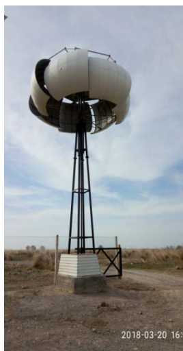
Figure 1 – “Torus” Wind Power Plant
